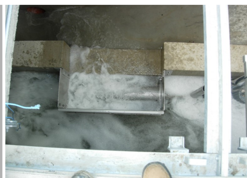
▲ Scouring action during the operational stage of the Pump Action Screen
