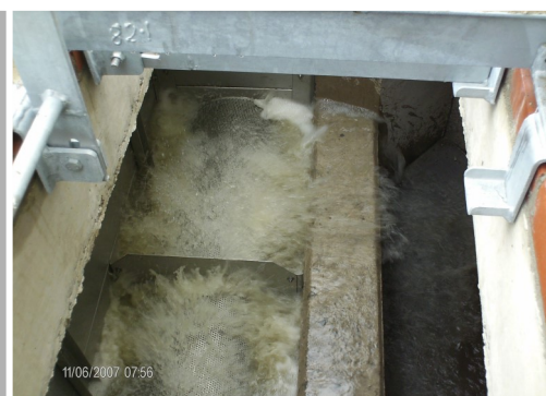
▲ Scouring action during the cleaning stage of the Pump Action Screen
