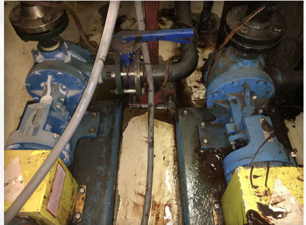
At Left: (O-Pro™ Barrier Seal pump with no leakage)
